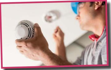
Specified types of sealed, long-life battery alarms or mains-wired alarms are permitted, with a maximum lifespan of 10 years.
